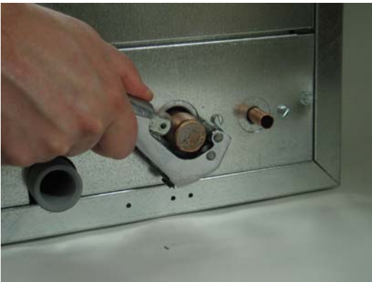
Cut end of connection as shown.
