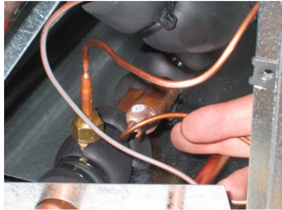
The thermal measuring bulb is placed as shown. It needs to be in contact with copper tube.
