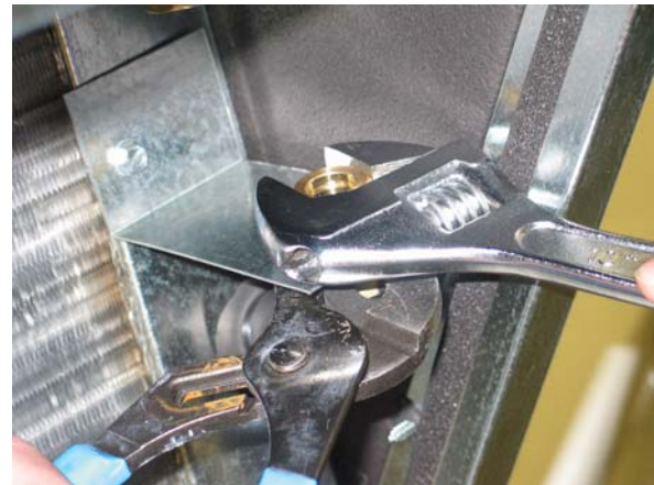
Remove nut as shown.
